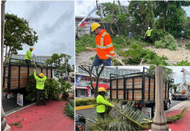
Tree Trimming & Debris Removal
