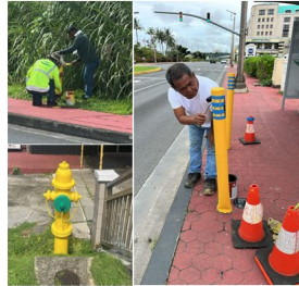
Repainting of Fire Hydrants & Bollards
